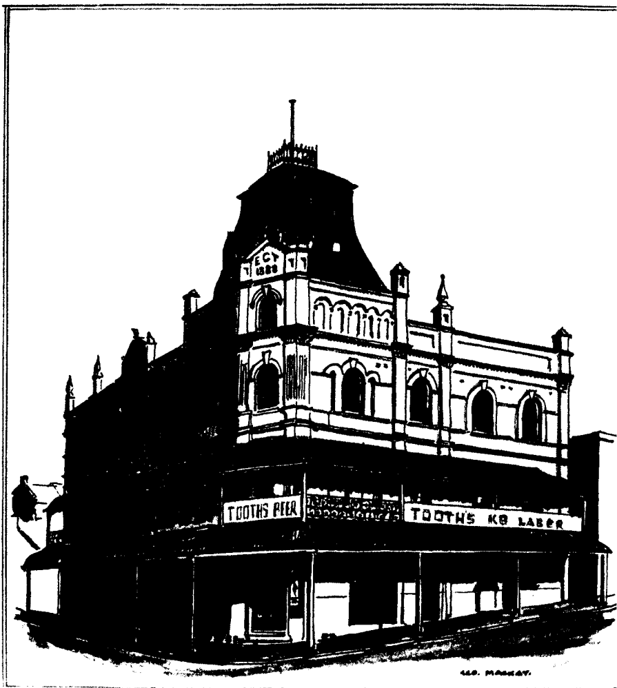
THE OLD HAROLD PARK HOTEL AT THE CORNER OF ROSS STREET AND WIGRAM ROAD. FORMERLY KNOWN AS THE LILLYBRIDGE HOTEL, IT WAS ERECTED IN 1888 AND DEMOLISHED IN 1959.
