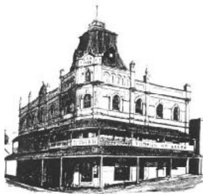
The old Harold Park hotel at the corner of Ross Street and Wigram Road. Formerly known as the Lillybridge Hotel, it was erected in 1888 and demolished in 1959.
