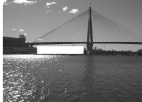
The proposed Slipway building would be the size of the white area. Photo: Bob Armstrong
