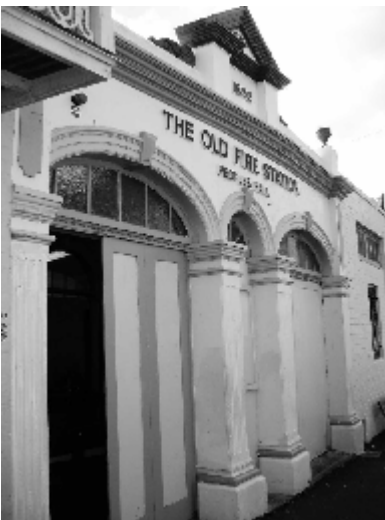
The Old Fire Station, Mitchell Street. Photo: Will Hayman
