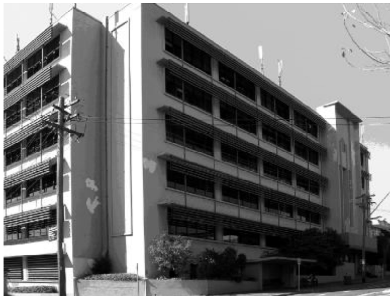
1947 Addition designed by David King. Photo: John Poulton
