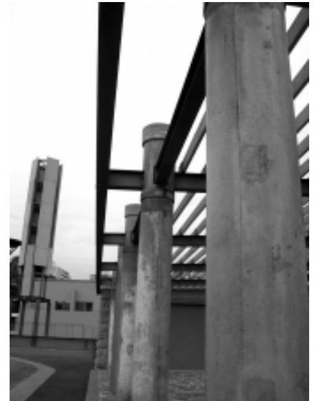
Photos clockwise from top left: Restored incinerator building with "chimney", original concrete columns that remained after the demolition of the workmen's sheds; view to Pymont, site of a larger Griffin incinerator; two details of art deco features on the main building.
