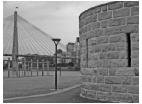
Sandstone "pillboxes" anchor the two lines of sheds.
