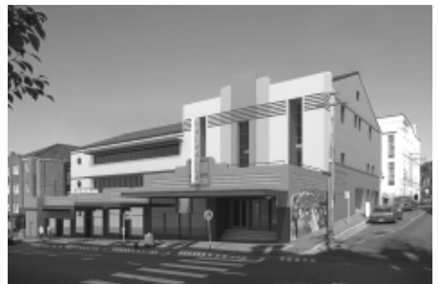
Artist's impression of the Valhalla with a new coat of render. Courtesy Prue and Mike Williams
