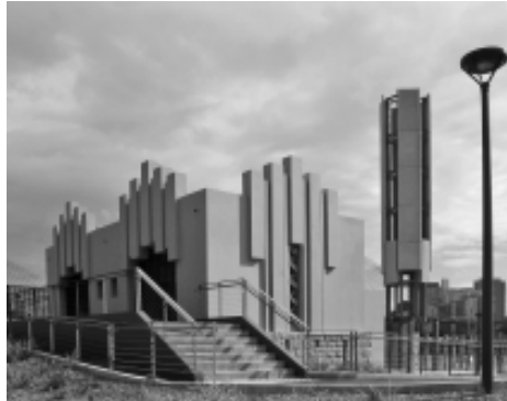
The restored incinerator at the end of Forsyth Street. Photo: Adrienne Kabos
