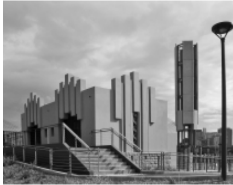
The restored incinerator at the end of Forsyth Street. Photo: Adrienne Kabos
