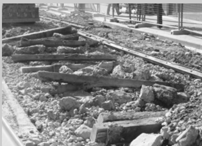
Sleepers revealed during the Glebe Point Road upgrade. Photo: Jan Wilson, 13 October
