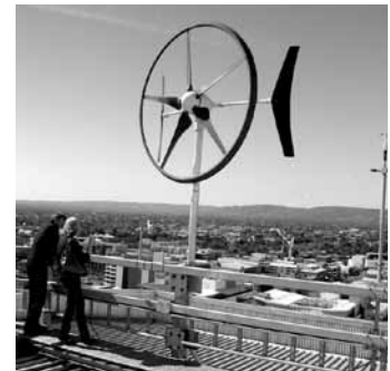
A small, roof-mounted wind turbine.
