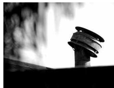
Tramsheds quietly decaying - a vent about to topple. Photo: Bruce Davis
