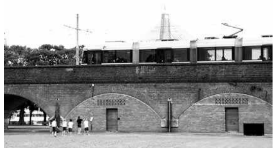
Two of the railway viaduct arches that will be opened up as part of the Wentworth Park upgrade.
