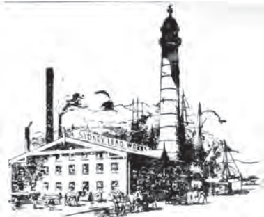
Sydney Lead Works, 1906
