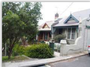
Palmerston Ave terrace row, off Keegan Ave.
