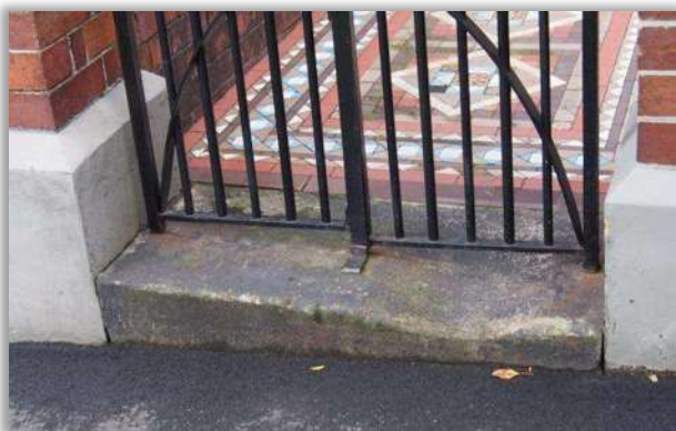
Telling a story : One example of the abrading effect of "the ceaseless tramp of feet" over a front step (for 114 years in this instance). (photo: Martin Lawrence)
