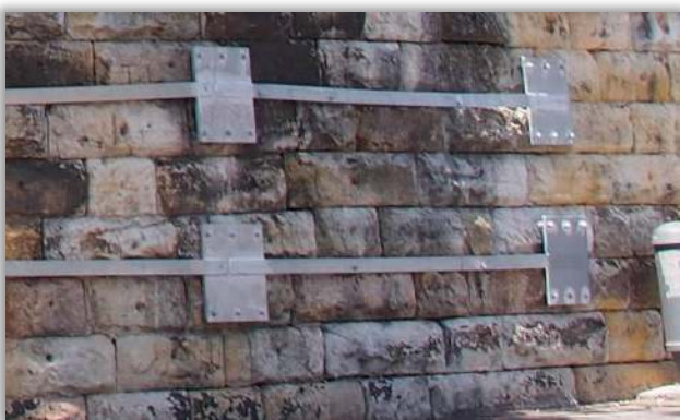
Close-up of stabilisation work at Forest Lodge School (image: Martin Lawrence)
