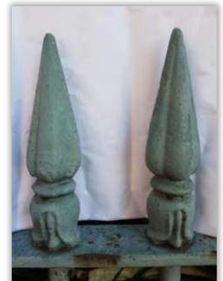
Fence at Emslee, Mansfield St (image: Peter Crawshaw)
