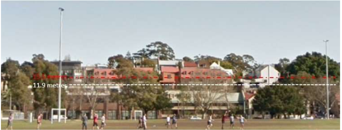
Figure 7 The white line shows the current non- conforming 11.9 metre building height in relation to the precinct and the red line shows the proposed 15.5 metre height.
