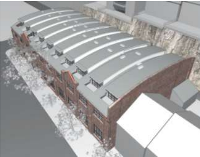
Figure 3 shows the 2005 attic insertions which retained the legibility of the curved roof
